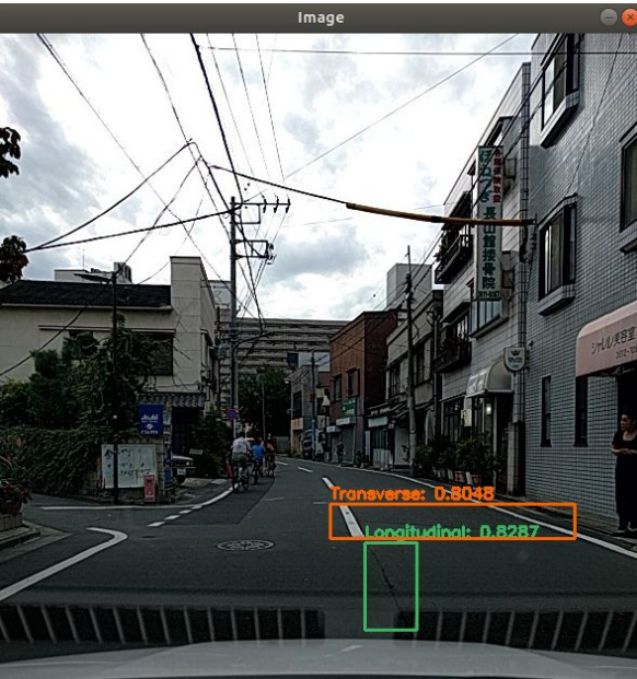
Figure 4. Algorithm performs transverse and longitudinal crack detection
